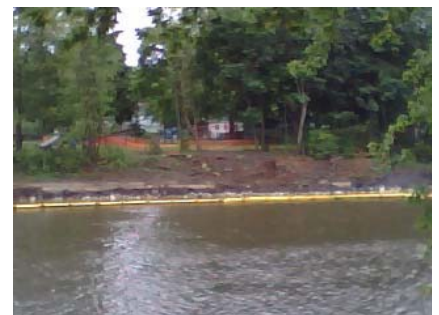
Riverbank Restoration in 015N
