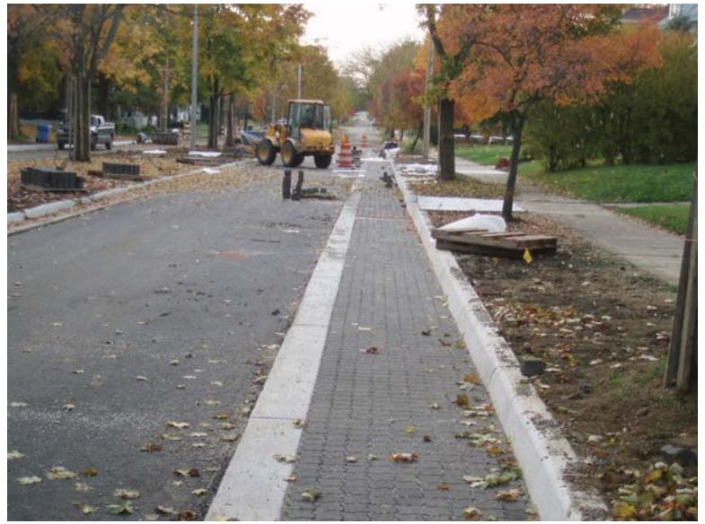
New Pavement and Pavers on Barnes in 034B
