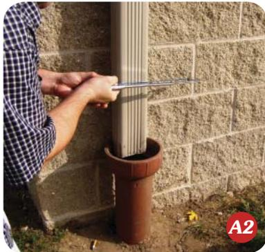
If you want the abandoned riser pipe closer to the ground, cut the pipe to ground level, being careful not to drop anything into the opening. Now that you have removed the downspout from the riser pipe, you need to permanently plug the pipe opening.
