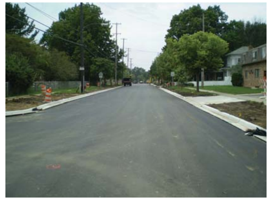
Base Paving on Willow in 015N
