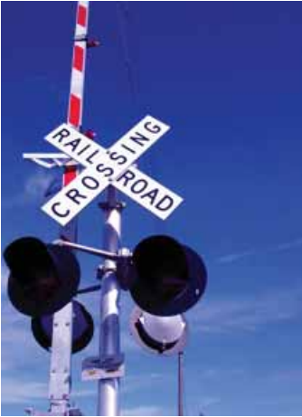
Improvements scheduled for this fall
