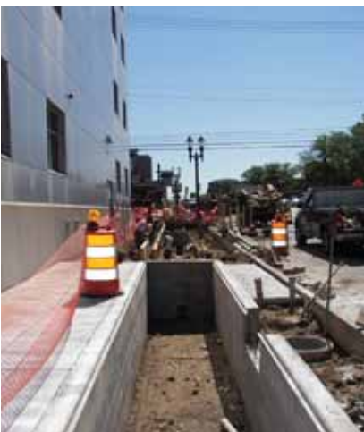
Rain garden construction
