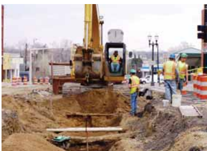
Excavation at Kalamazoo and Washington
