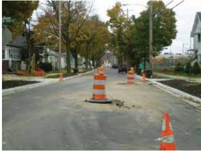
Manhole work on Ballard
