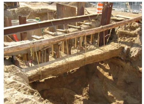
Electric and Telephone Supports at Washington and Allegan
