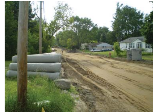
013NE Storm Sewer Ready for Installation on Howe near Turner
