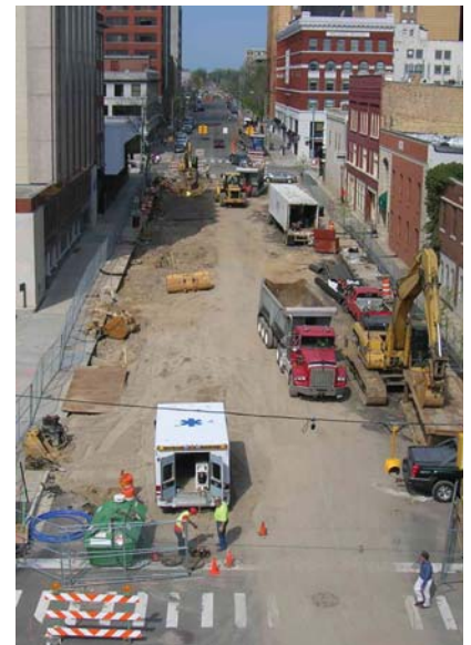
Construction on Allegan
