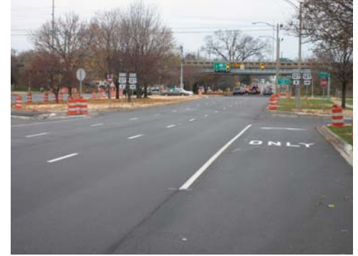
Michigan Avenue Resurfacing
