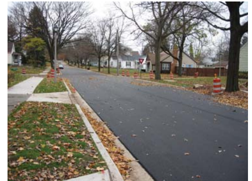
Resurfacing on Park
