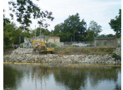
Riprap Installation to Restore River Bank in O15N
