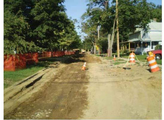
Barnes Under Construction in 034B
