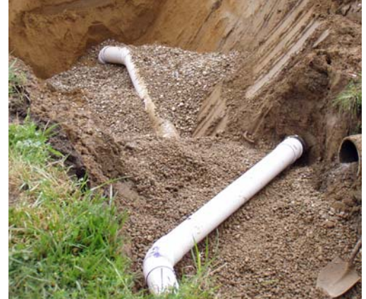
Sanitary Service Lateral Installation in 045
