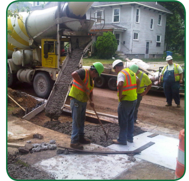
Concrete restoration on Wisconsin
