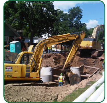
Sewer installation on Oakland and Chicago
