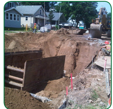
Sanitary and storm installation on Oakland at Wisconsin
