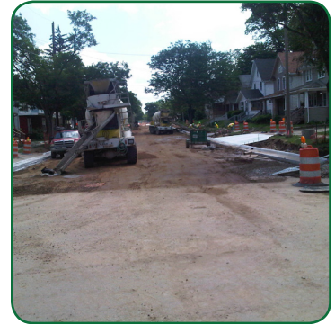
Concrete restoration on Oakland, between Pine and Walnut
