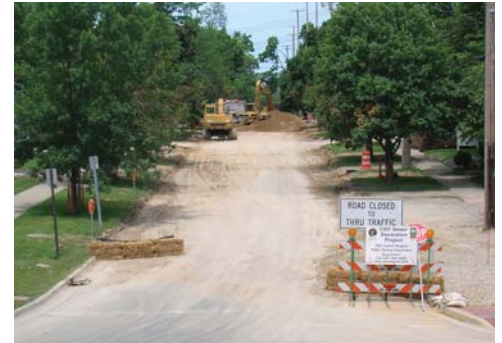
Construction on Chestnut
