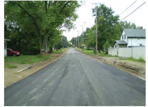
013NE New Pavement on Orchard Glen
